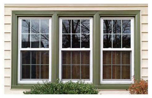
An external window or door is classed as a "controlled fitting" under the building regulations and as a result of this classification these regulations set out certain standards to be met when such a window or door is replaced.
